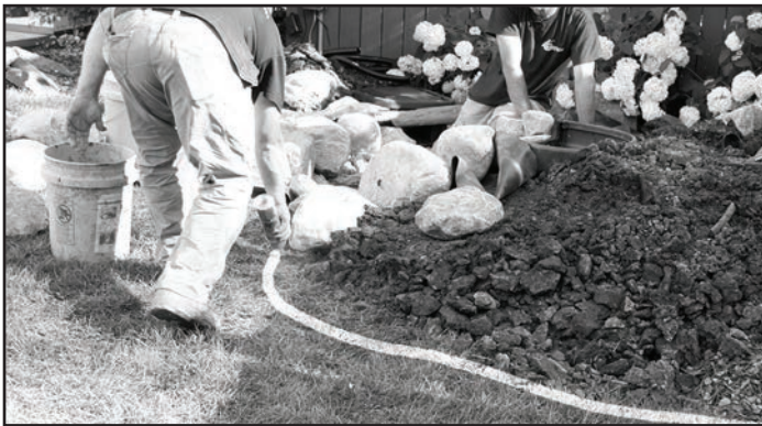
Trim off any excess liner.
